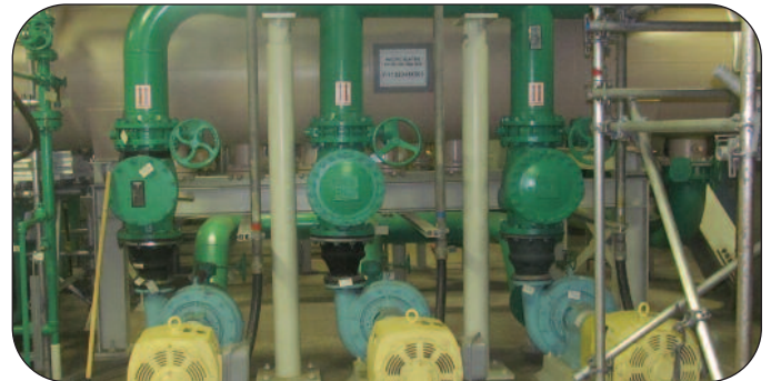
Thorburn's 42HP-CR Concentric & 42HP-OR reducing expansion joints installed in pumping station at the OPG Pickering nuclear reactor
