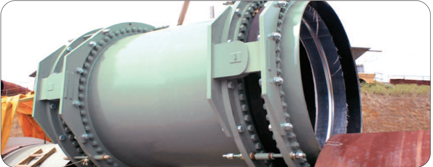
Thorburn's 42HPWX-H 1830mm (72") Universal Hinged Expansion Joint Being Installed at a Nicaraguan Geothermal Power Plant
