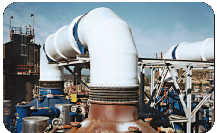
Quantity of 12 Thorburn 62HPW 900mm (36") Rubber Expansion Joints installed on a GRP piping system at a sulphuric acid plant in Baja Mexico
