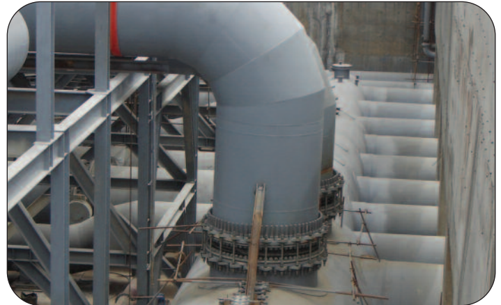
Quantity of 36 Thorburn 42HPW 1200mm (48") Rubber Expansion Joints installed at a power plant in the middle east
